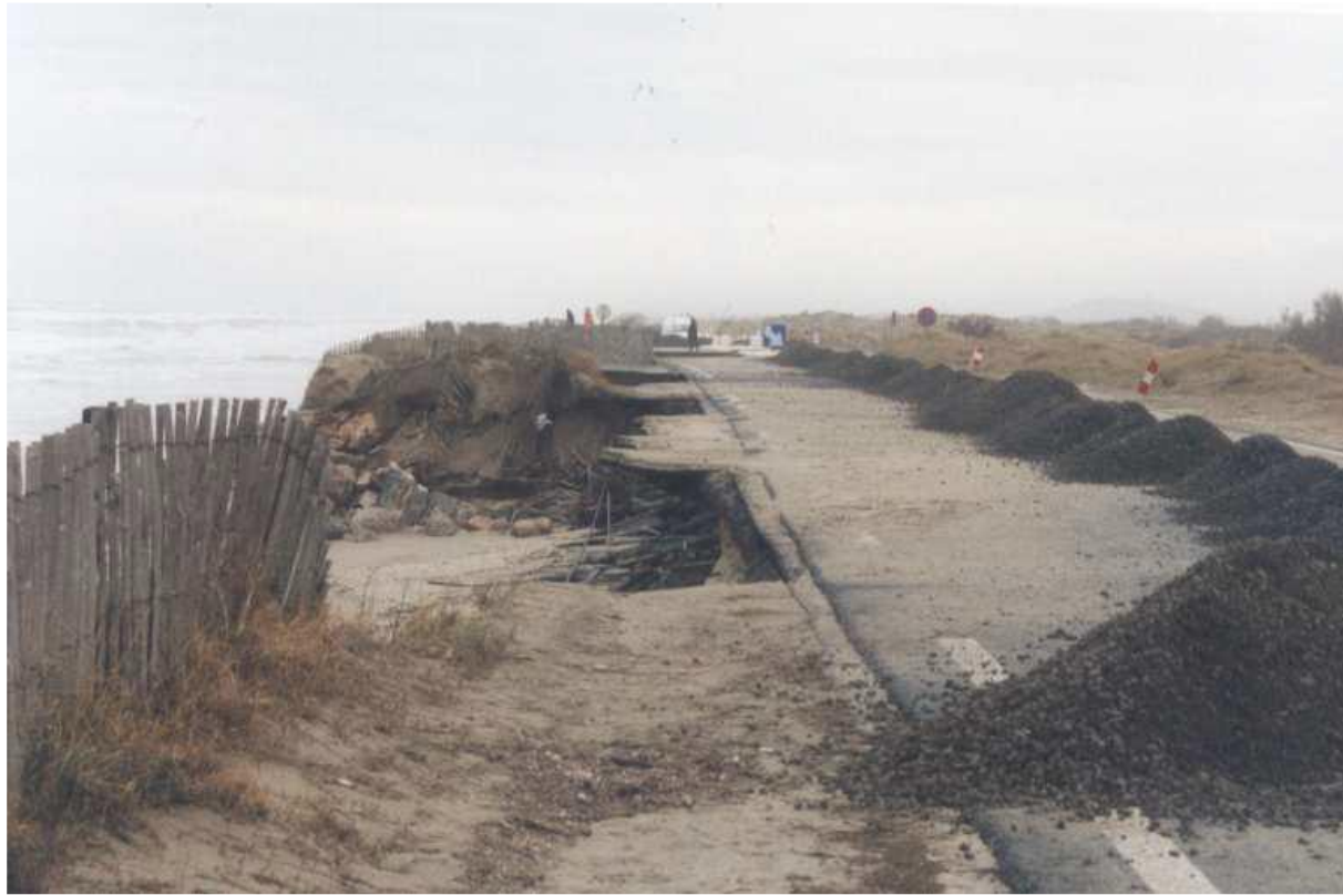
Pict. 1 : Recurrent erosion impacts on the coastal road
