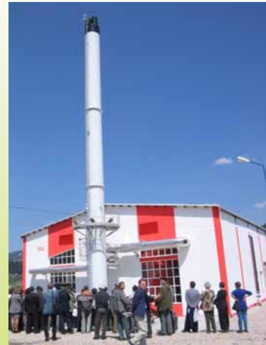
Vatra Dornei Biomass District Heating Plant
