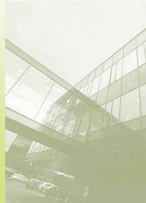
Head Quarters at Nupark Office Complex
